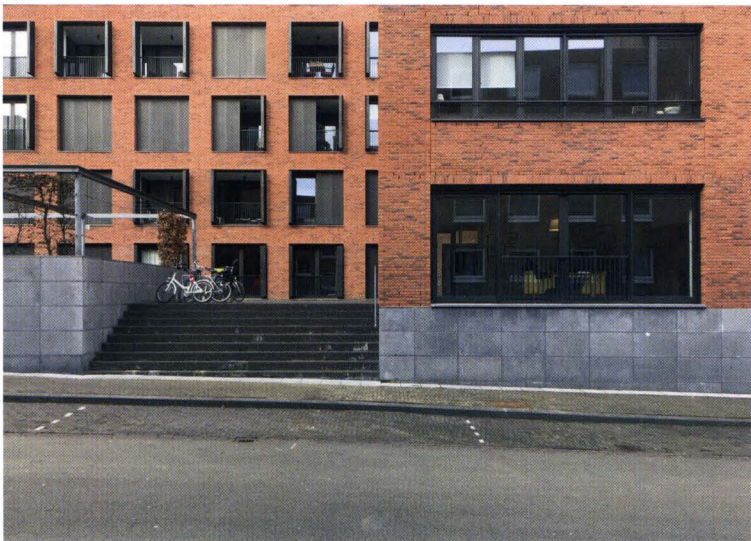
Appartementengebouw (A, links) en rij praktijkwoningen (C, rechts) Residential building (A, left) and terrace of dwellings with work space (C, right)
